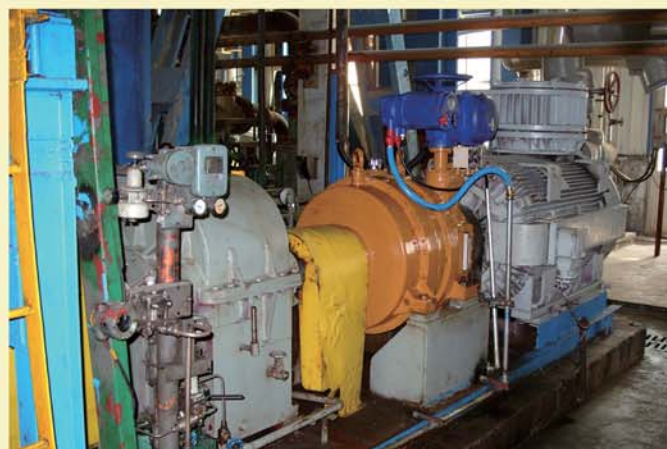
可调液力变矩器在乌石化使用现场 Adjustable hydraulic torque converter at the job site of Wulumuqi Petrochemical
